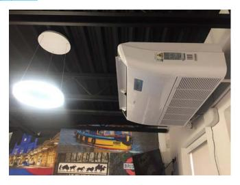
The equipment required had to be compatible with the chosen refrigerant; R-32. Climalife was looking for a number of split systems for individual offices but also needed a number of larger 16-18Kw multi split systems for the larger open plan areas.
